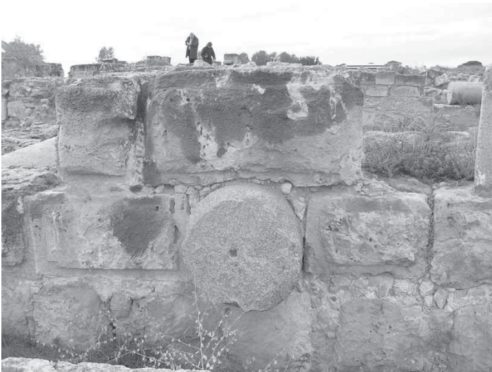
Fig. 13: Kato Paphos, Saranda Kolones Castle, detail of marginally drafted masonry [M. Olympios].
